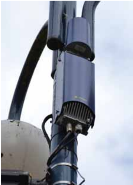
Figure 6: Small cell deployment on a lamppost
